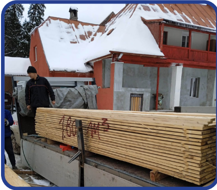
A new roof for St. Anton's
